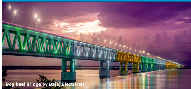
Bogibeel Bridge by Bajaj Electricals
