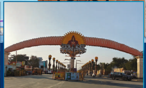
Surya Stambh lighting with Philips Uni facade
